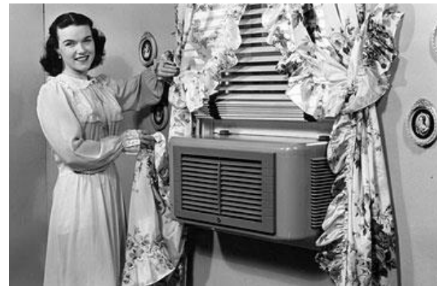
Fig 2.5 Window planted Air conditioner
