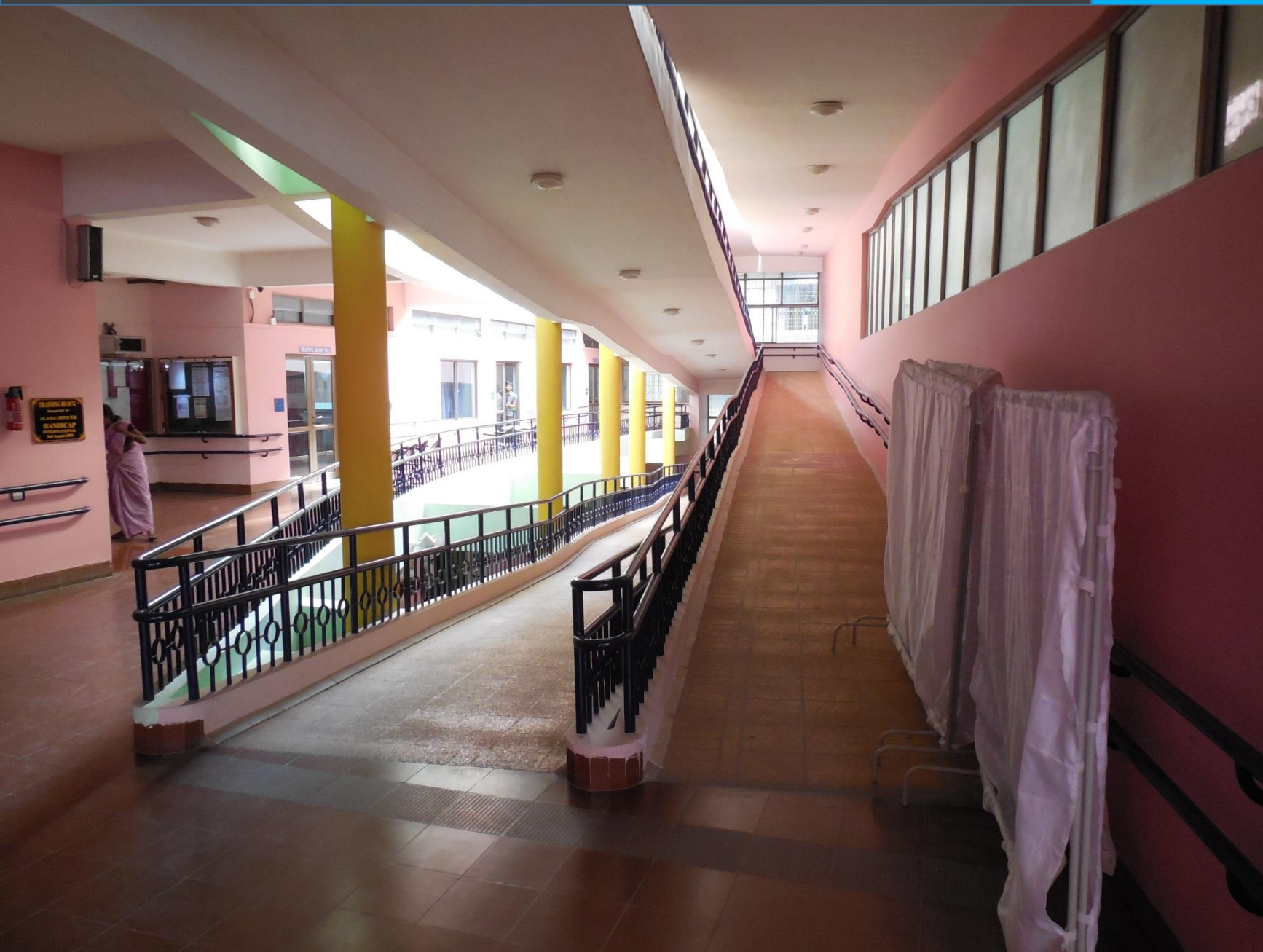
Wheelchair ramps and railings in administrative block
