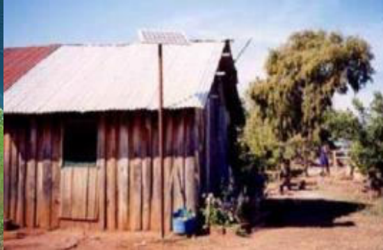
50 Wp PV lighting system installed in Talayotes, Moris County, Chihuahua.
