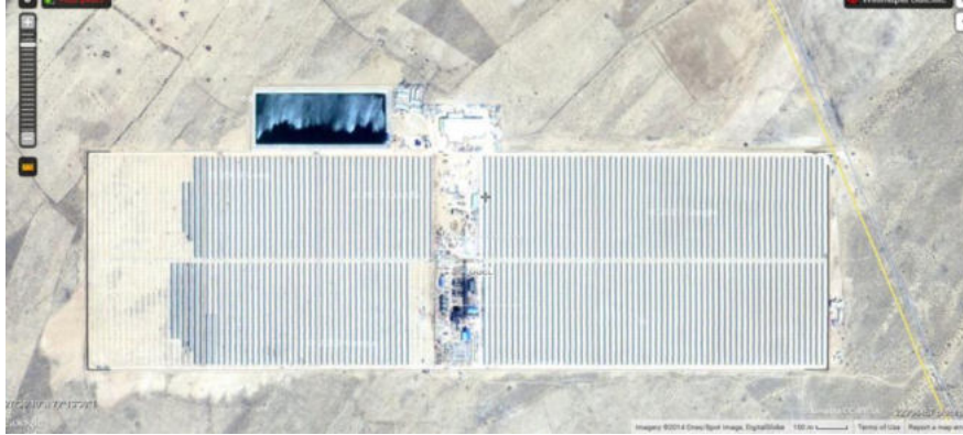
Fig. 8 Godawari Green Energy Concentrated Solar Power Plant, Rajasthan
