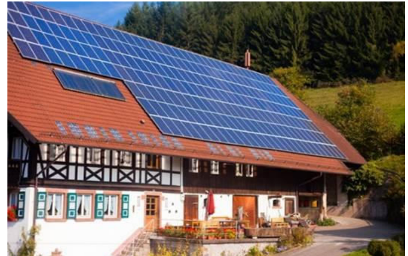
Fig. 13 Solar panels on rooftop in Bavaria, Germany
