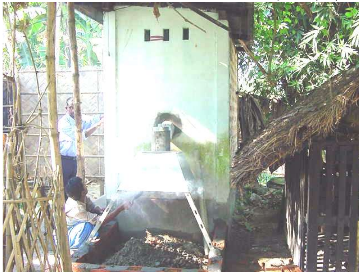
Smoke chamber built being modified as per requirement
