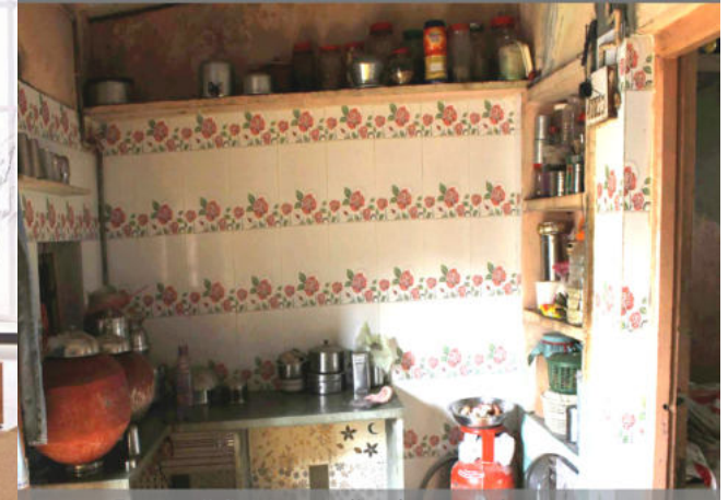
Fig.15 Wall finish in Indian low cost houses
