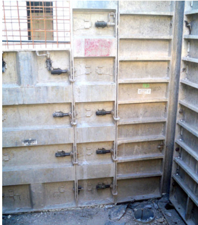
Fig.24 How shutters are joined together
