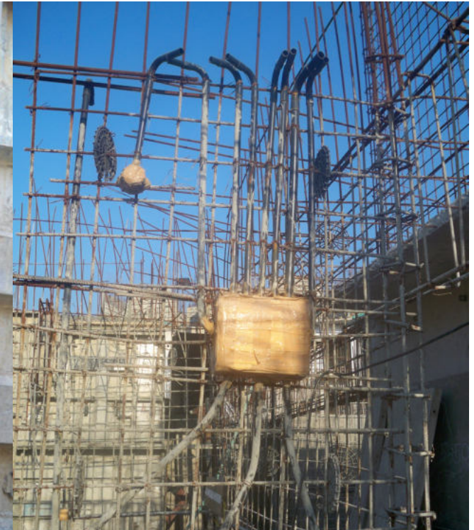
Fig.27 Placing switch board and pipes
