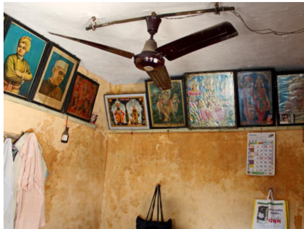
Fig.19 Wall treatment and electrical wiring
