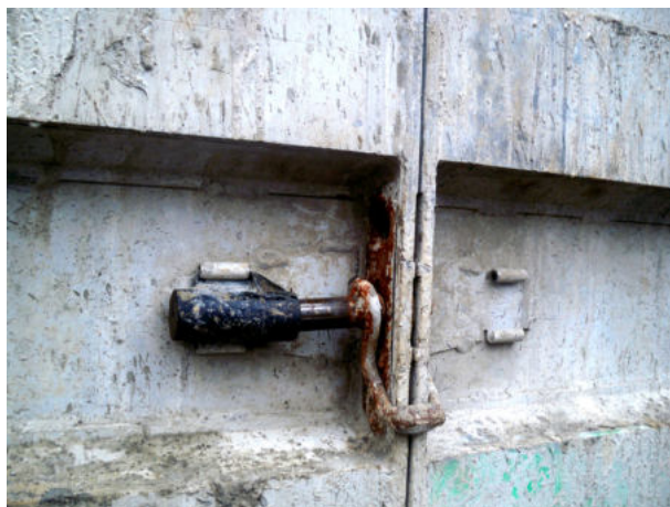
Fig.28 Detail of joining shutters
