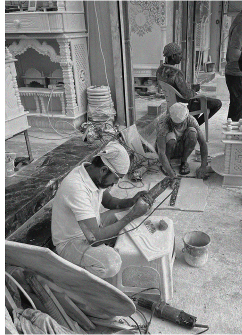
Fig 13.2: Encroachment Outside Workshop
