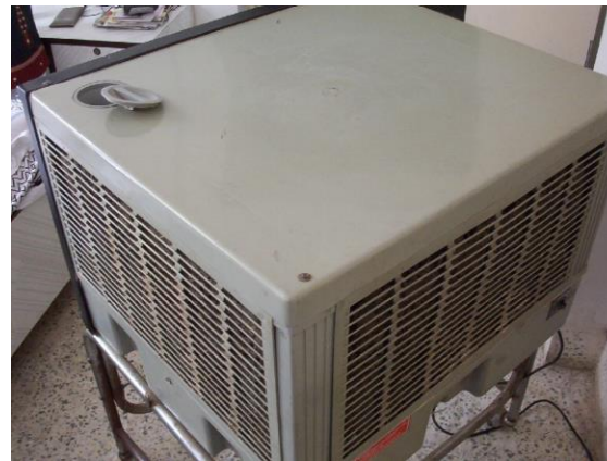
Window unit therefore openings on all three sides
