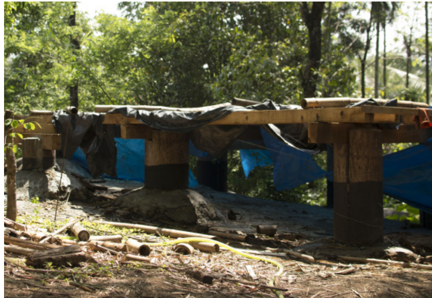
Fig 37 - Palm and concrete structure for base construction
