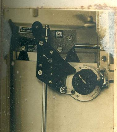
weights. It can be adjusted and locked in any desired position for height and angle by means of the height variation mechanism and the hand lever.
