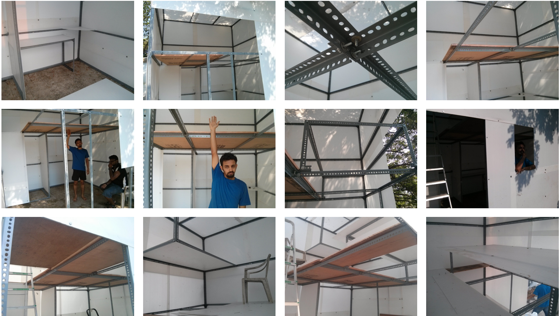
Fig 37. Building life-size model frame (contd.) - construction of upper level
