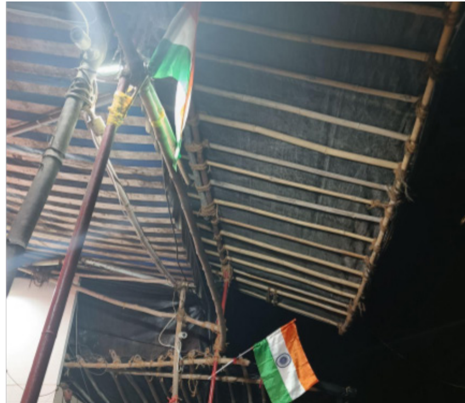
Wooden scaffoldings for rain protection in Khau Gali
