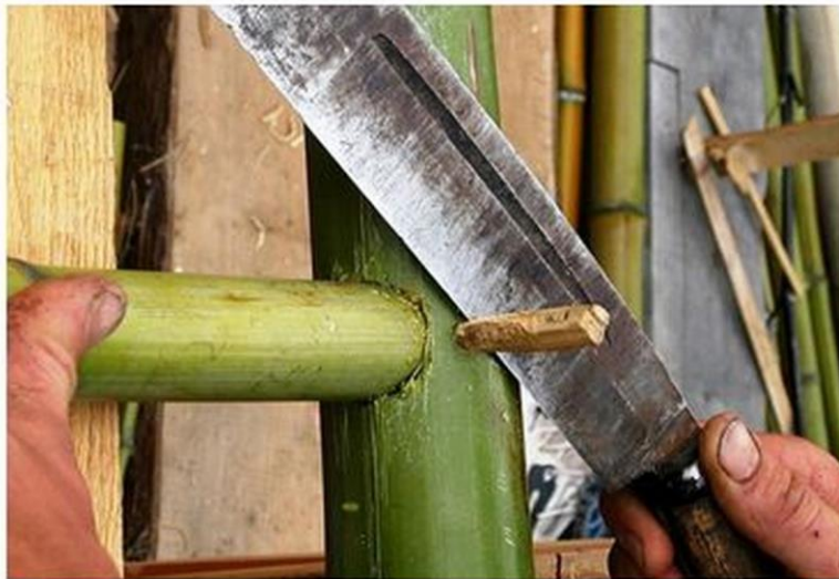
positive fitting bamboo connections
