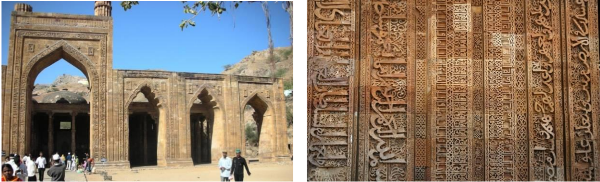
Figure 2.135 - Adhai - Din Ka- Jhonpra in Ajmer, Rajasthan
