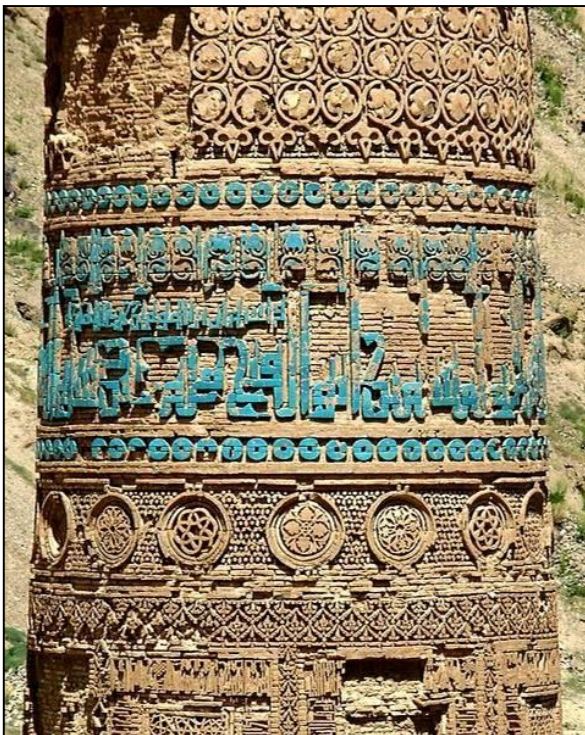
Figure 2.124 - The Minaret of Jam is located in the Shahrak District, Ghor Province, The 65 metre high minaret, was built in the 1190s, entirely of baked-bricks.
