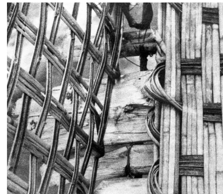
Detail of side wall and floor of walkway, of a bridge. Strips of various types are used for wall and floor.
