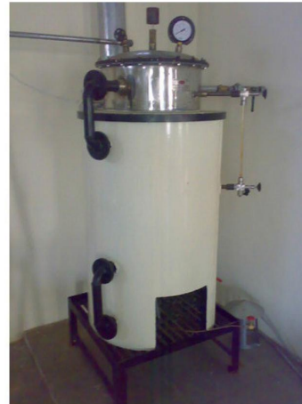
Fire wood steam boiler
