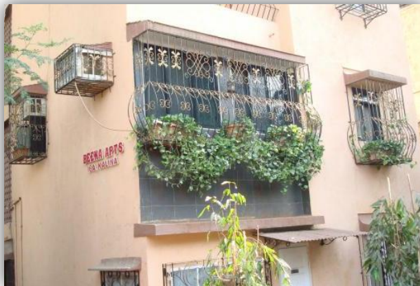
Fig.5 Apartments with security grills in mumbai
