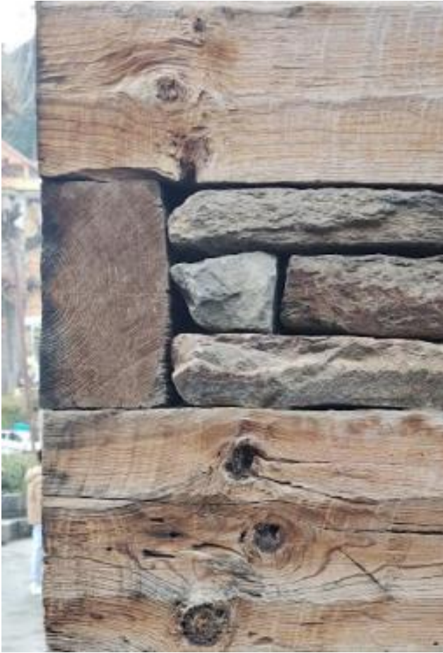
Fig 19 : Joinery details in Kath Kuni Design.
