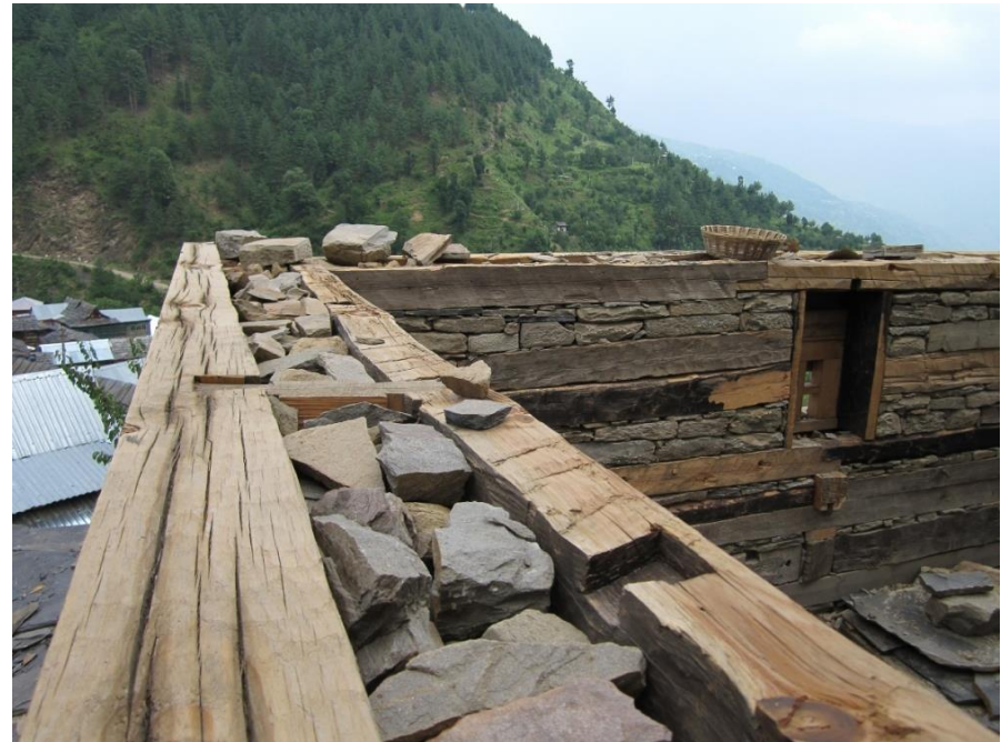
Fig 38: Traditional Kath-kuni wall laying pattern (source: sahapedia.org)
