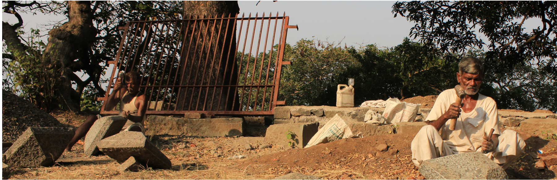
> Workers on Conservation work. Sculpting the rocks.
