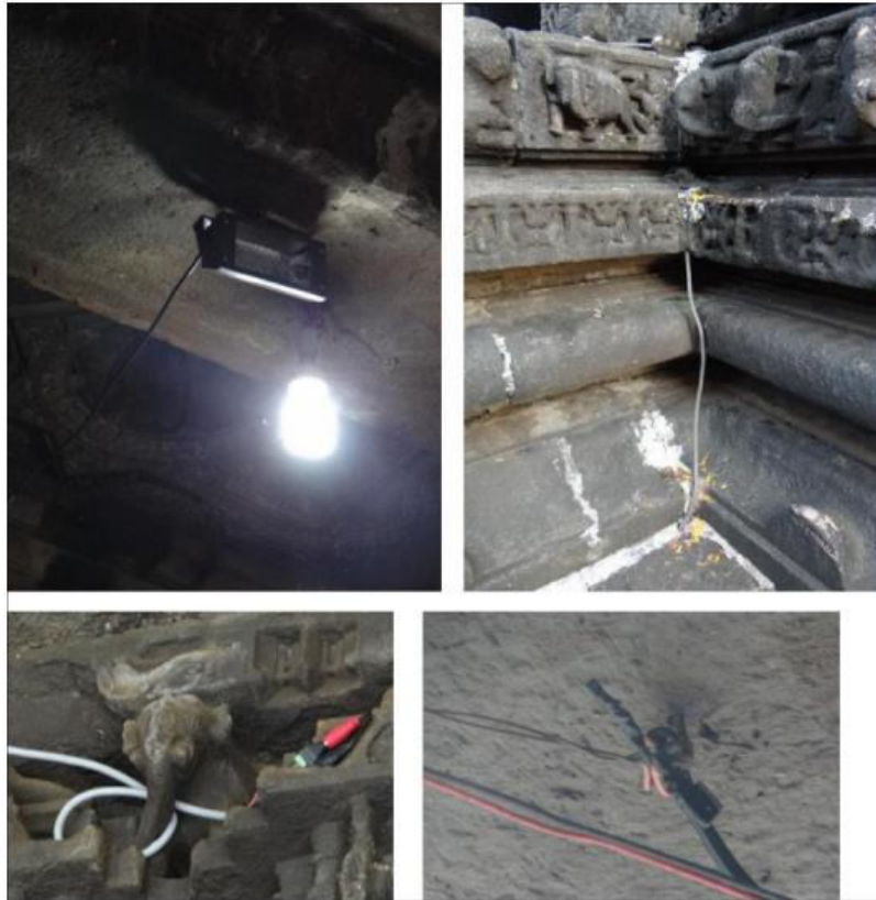
Wiring, fixtures and power supply units, Ambarnath temple
