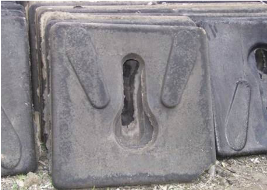
Figure 3 Molded slab of the Arborloo toilet type (Source: http://faculty-staff.ou.edu assessed in August 31/2013)
