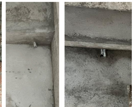
Fixed positions for tube/LED's (cannot be change after the location of the light is finalized)
