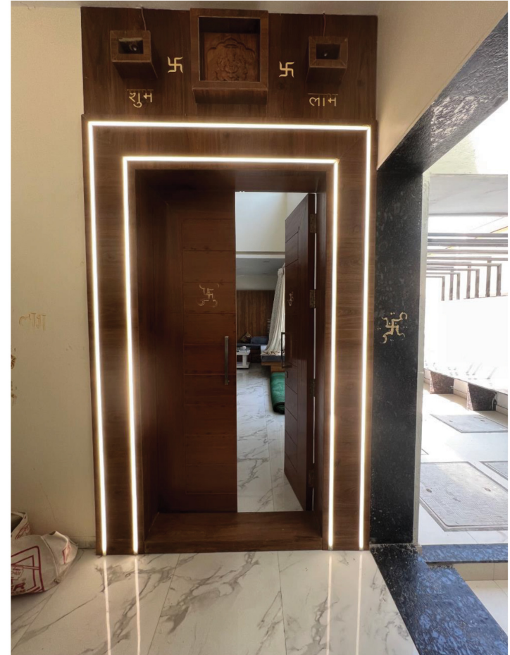
Entrance with LED Strips ( on wooden door frame)
