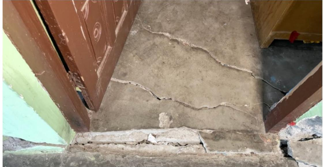
Fig 2.9 Issac, R., The cracked plinth of house marked for demolition. Joshimath. 2023.
