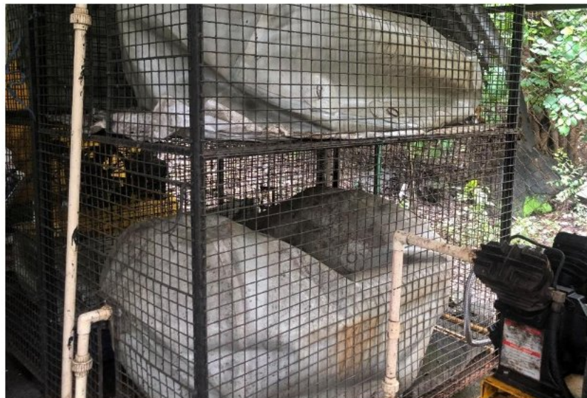
Figure 15 - Mixing tank, digester, storage tank
