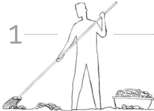
1 Scraping the waste from the top surface
