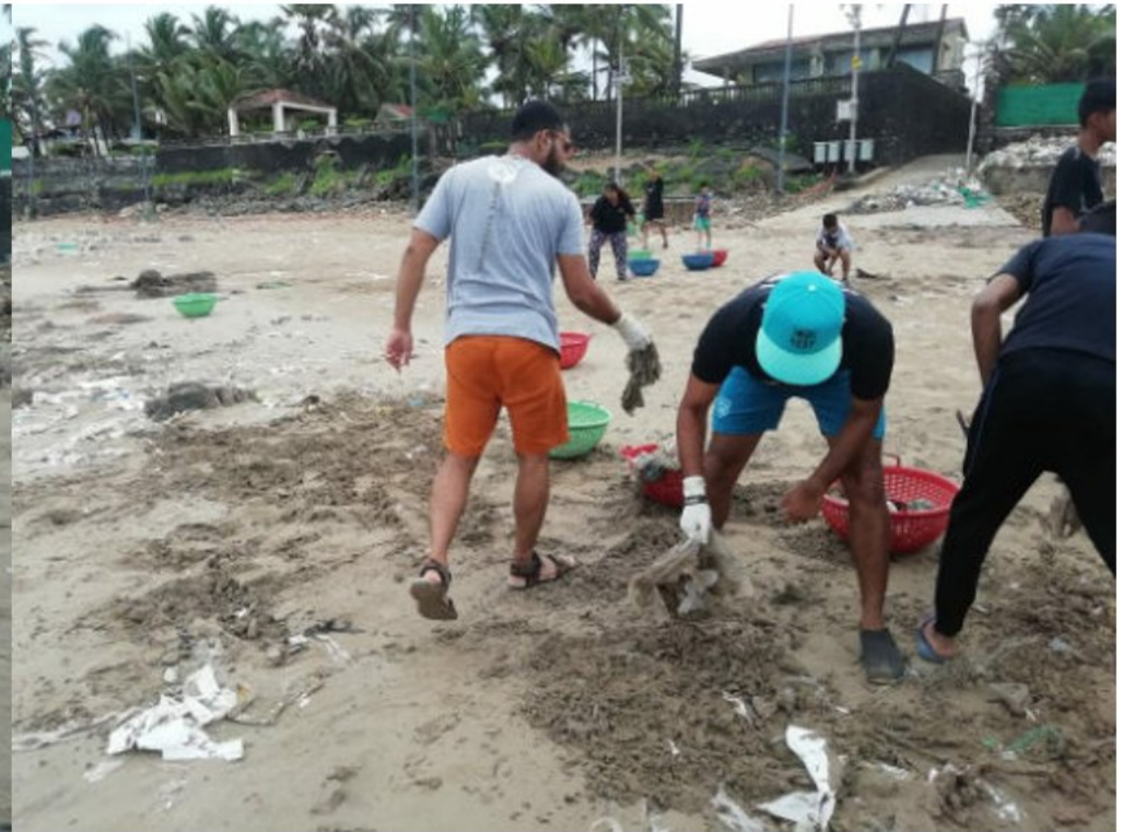
Image 32: A surprising amount of plastic sheets filled with sand were found underground
