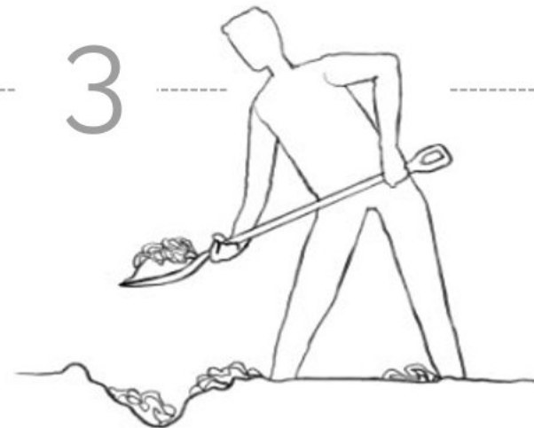
3 Digging the surface for partially sunken waste removal
