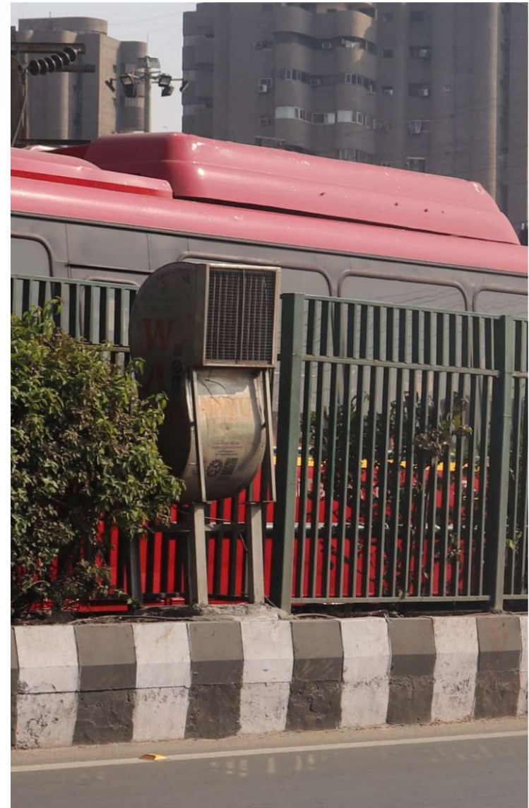
WAYU air purifier installed on the divider of the road.
