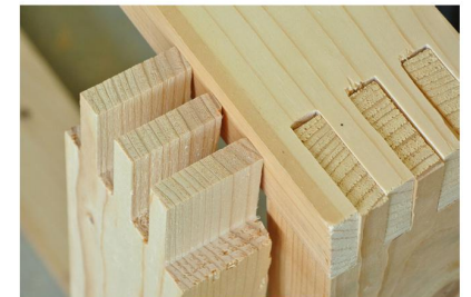
fig 2.33 Through-Dovetail joint
