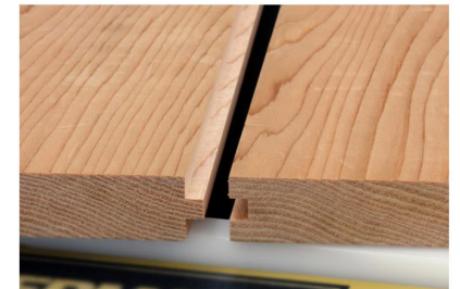
fig 2.34 Tongue and Groove joint
