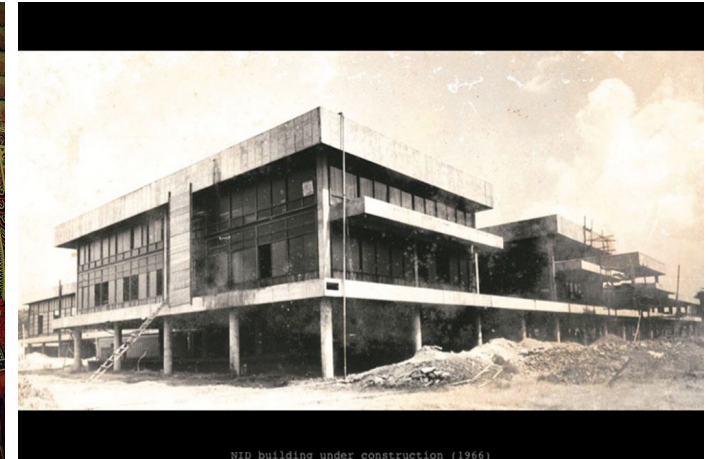
NID building under construction.
