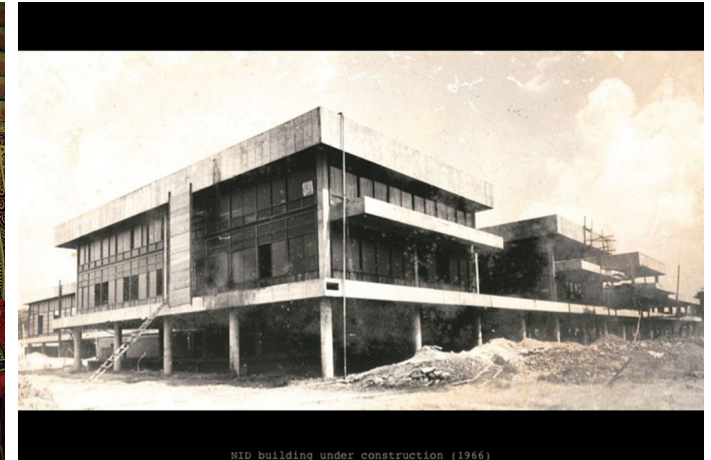
NID building under construction.
