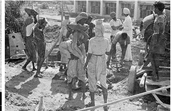
Construction workers handling the Ghamela on site.
