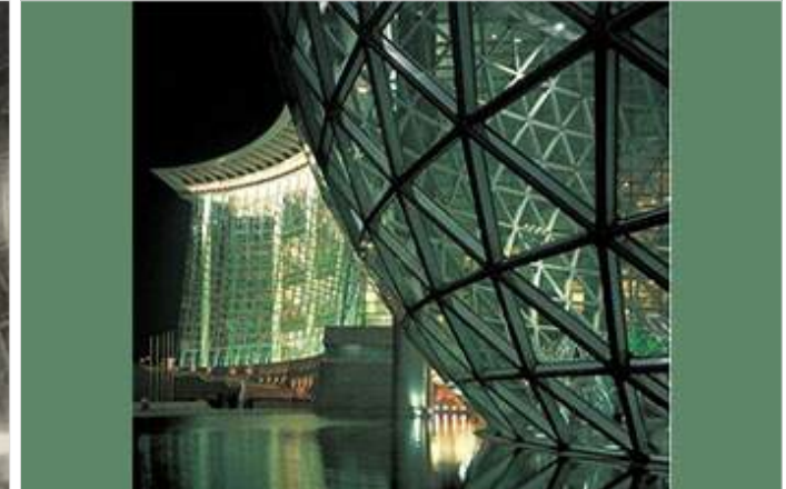
Duralumin in a dome construction. (Image source)
