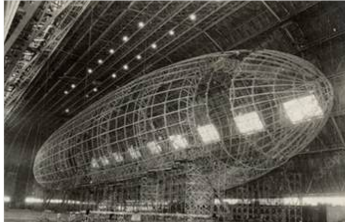
Duralumin in airship body construction. (Image source)
