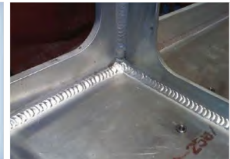
T Butt welding in a structural frame. (Image source)
