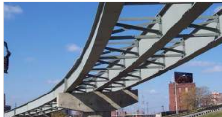
Girders using HRCA Plates.
