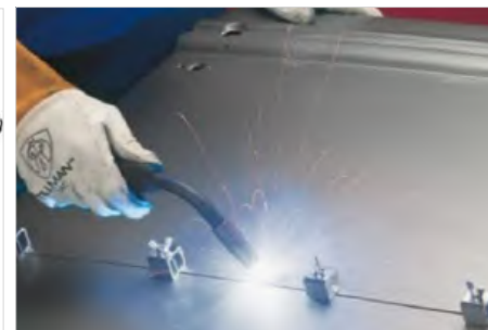
Butt weld in progress.
