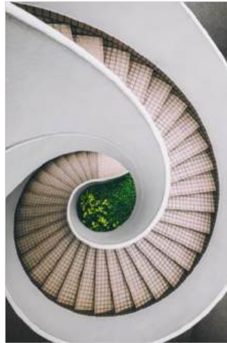
Staircase with perforated Metal steps. (Image source)
