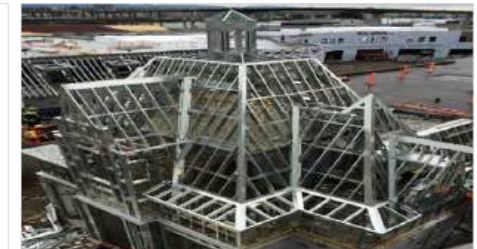
Construction. (Image source)
