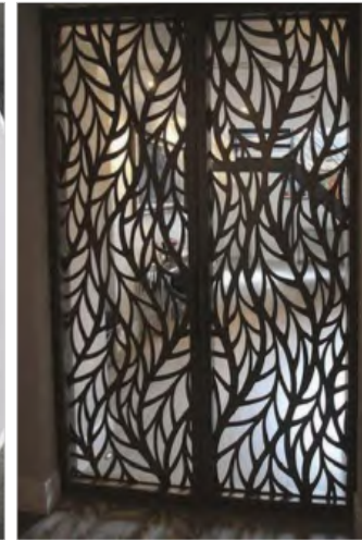
Laser cut seet steel door panels. (Image source)
