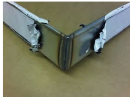
Typical corner welding. (Image source)
