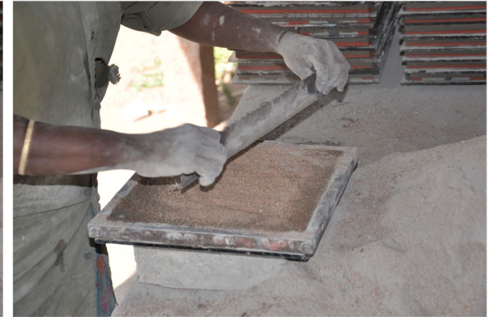
Extra mortar is removed with the help of blade.
