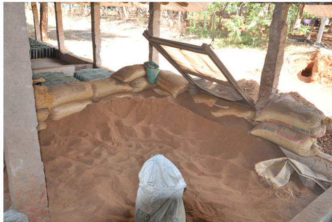
Local sand is sieved/ filtered to remove unwanted material.
