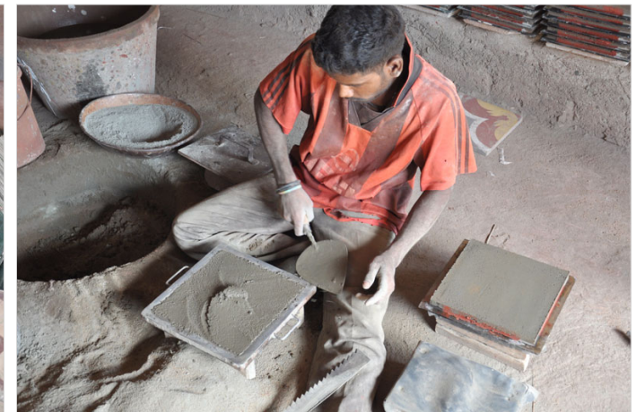
Spade is used to properly spread the cement in the frame.
