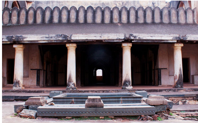
Front view of the Rangeen Mahal.
