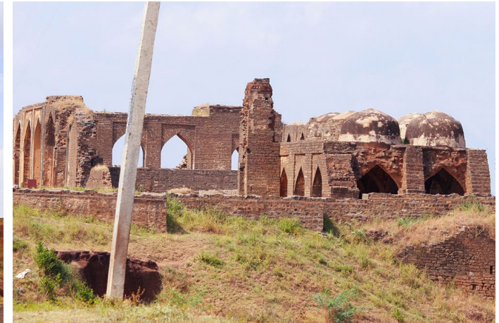
Left end view of the structure.
