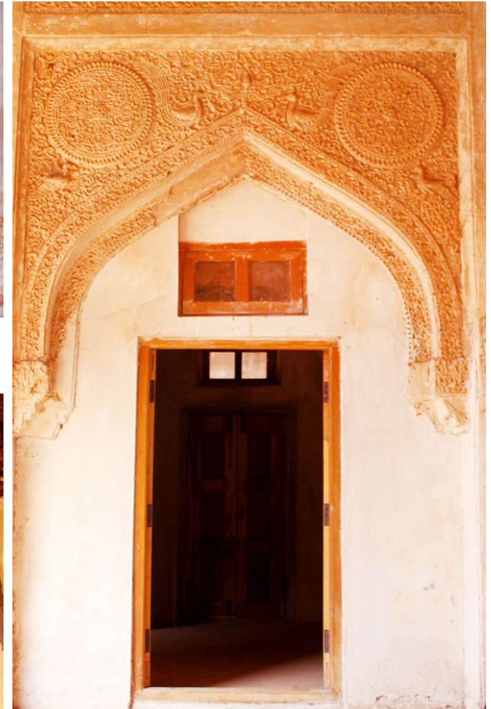
Beautiful mural work on the door arch.
