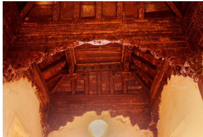
The Rangeen Mahal roofs.
