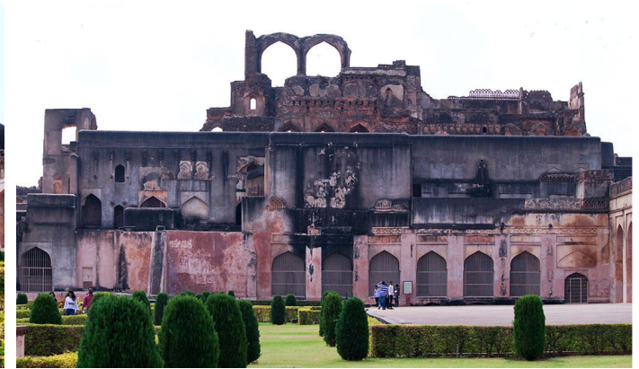
Front elevation of the Takht Mahal.
