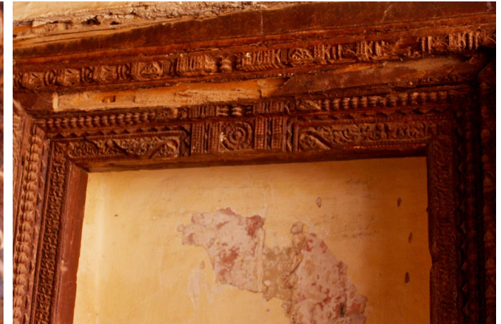
The wooden frame of the Mahal door.
