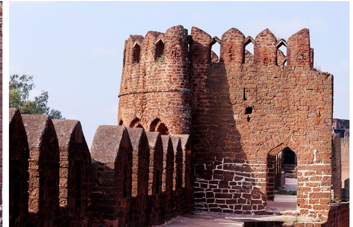
The top position of the watching tower.
