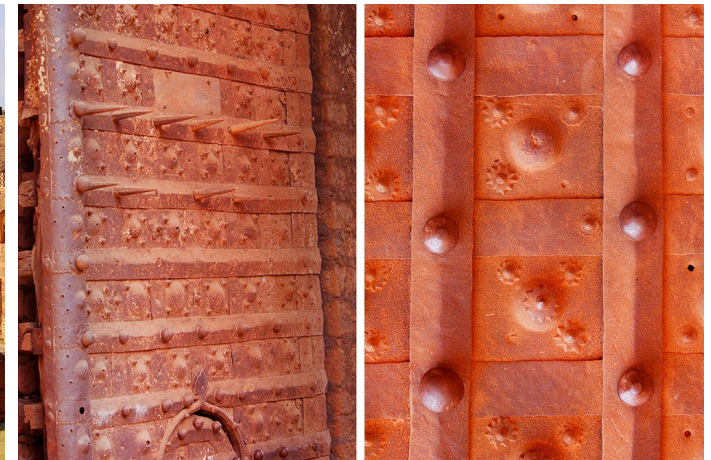
Front gate door.
