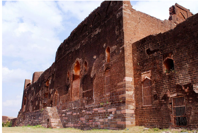
View from the interiors of the old fort.
