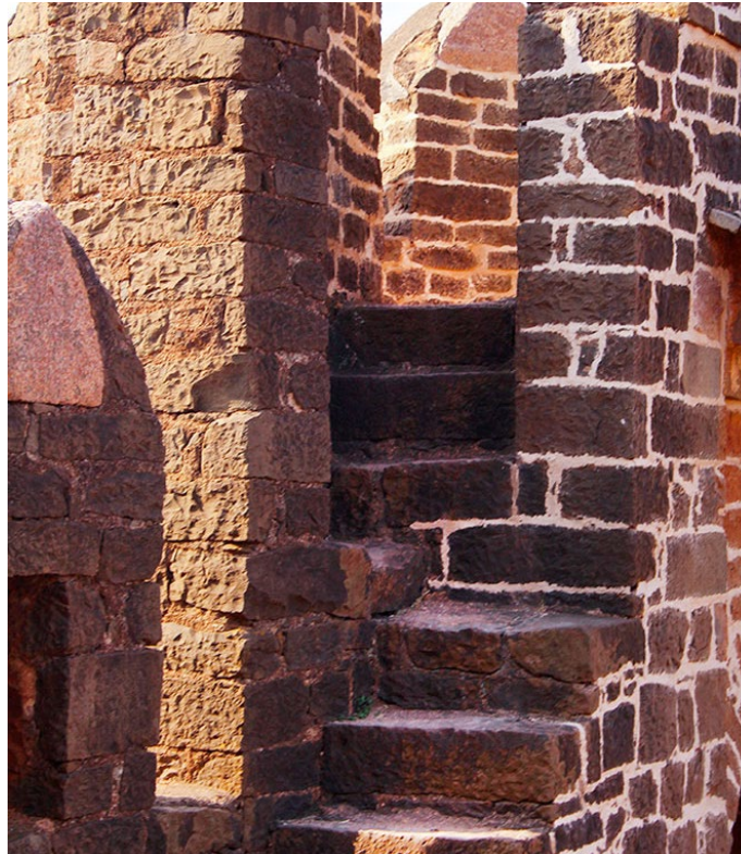
The steps of the watching tower.
