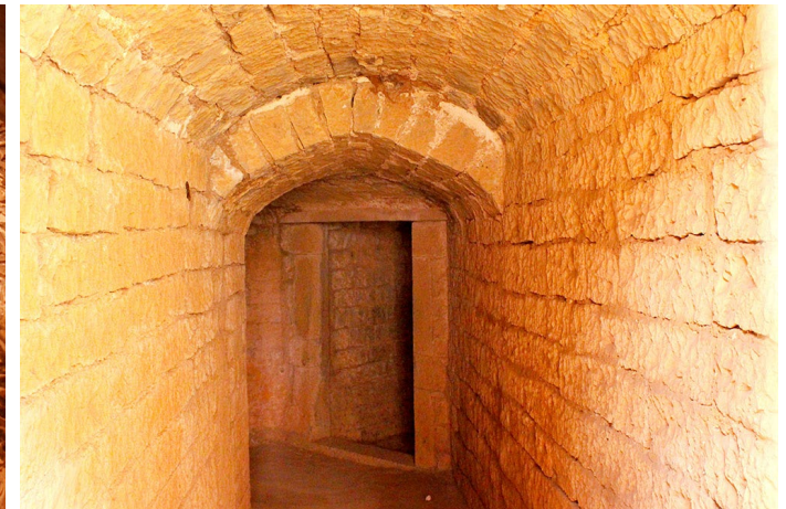
The basement path of the fort.
