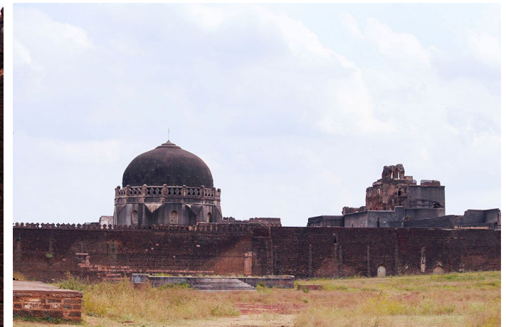
Dome-shaped building structure in the interiors of the fort.
