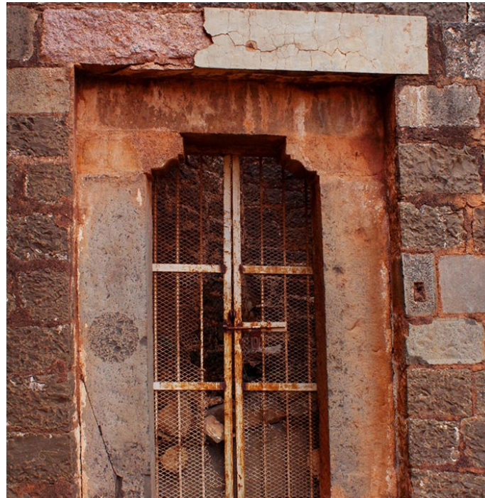
The door with a stone frame.
