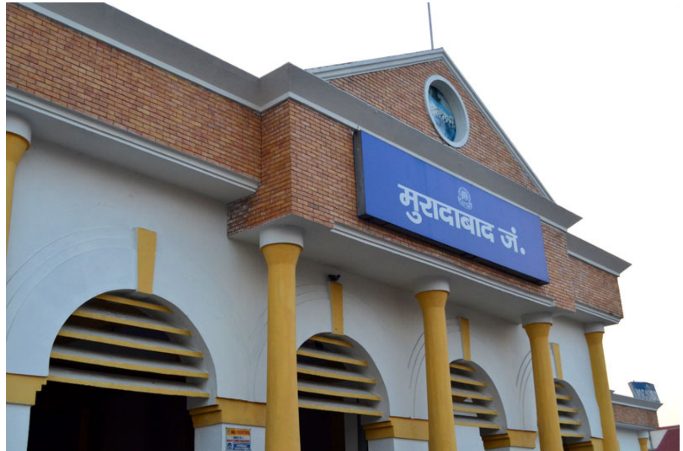
Outside Moradabad railway station.
