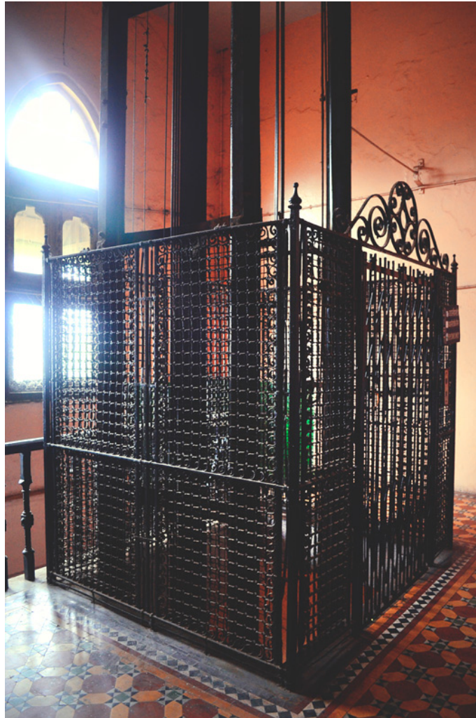
British era lift is still used by the office.
