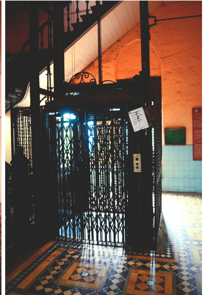
British era lift is still used by the office.
