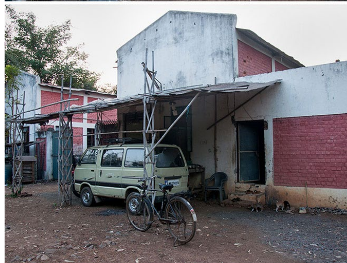
The outside view of the Vedha India factory building, also known as the Institute of Village Interments Development for Artisan, is based in Nagpur.
