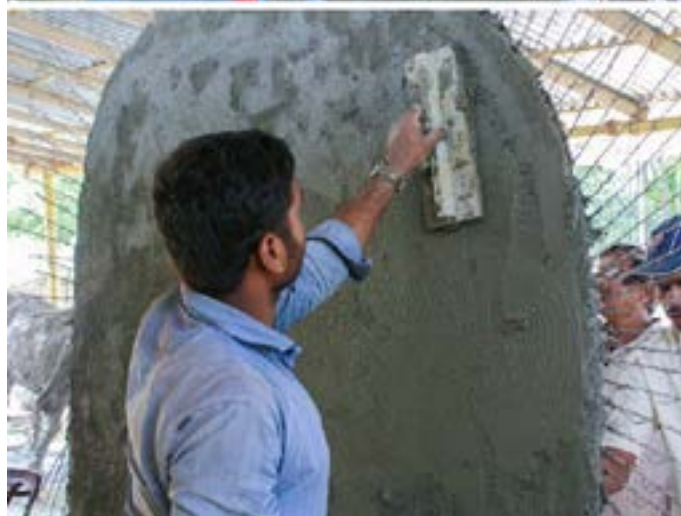
The mesh is covered by a layers of cement.
