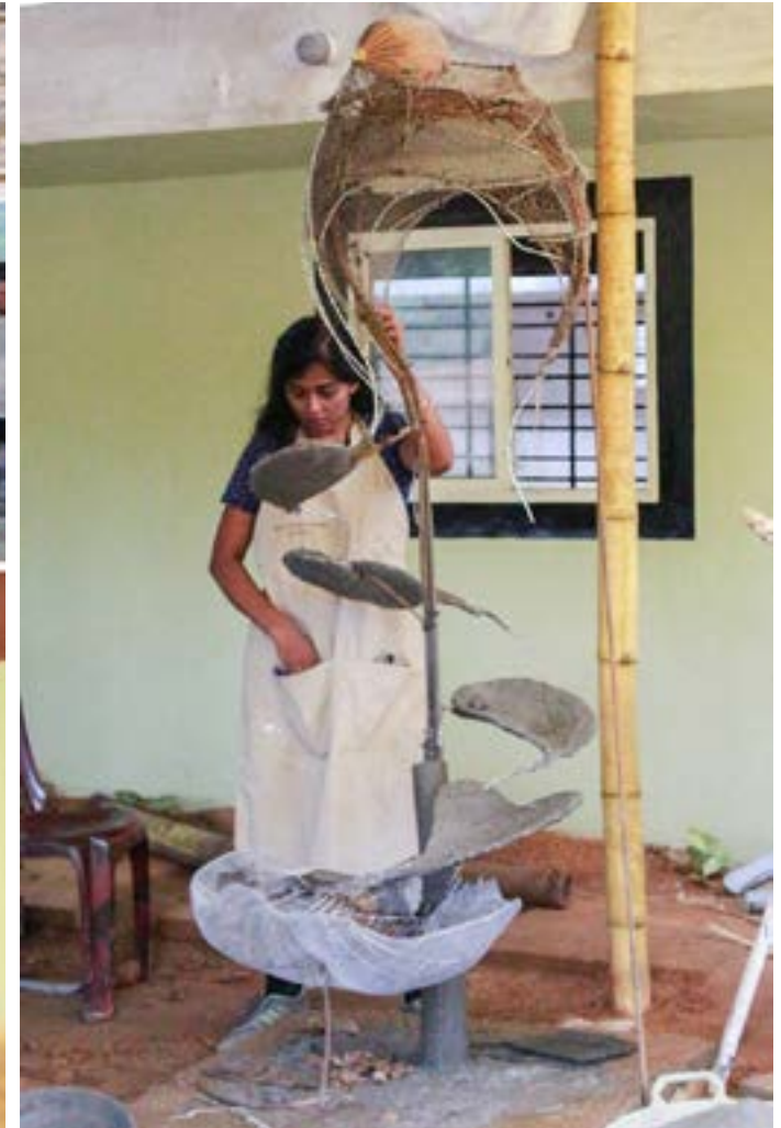
Mesh is covered all over and cement is applied over to make it stronger.
