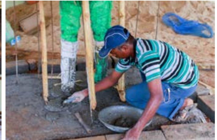
The skeleton of the sculpture is strengthened by a thick layer of concrete.
