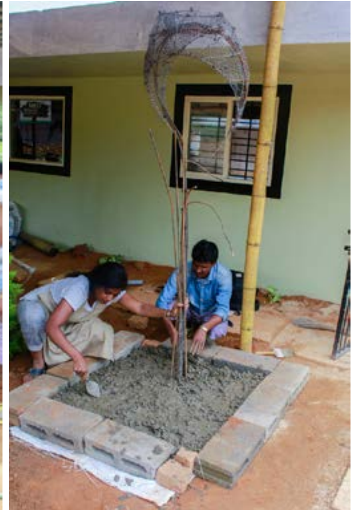
Strong base is made by using concrete.
