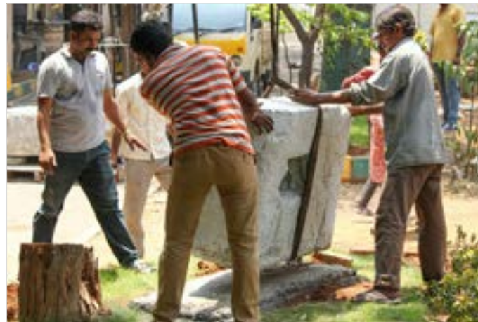
Initially bottom portion is placed on the pedestal.
