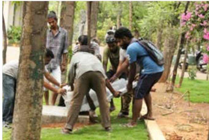
Installing Buddha sculpture on the pedestal made up of concrete.
