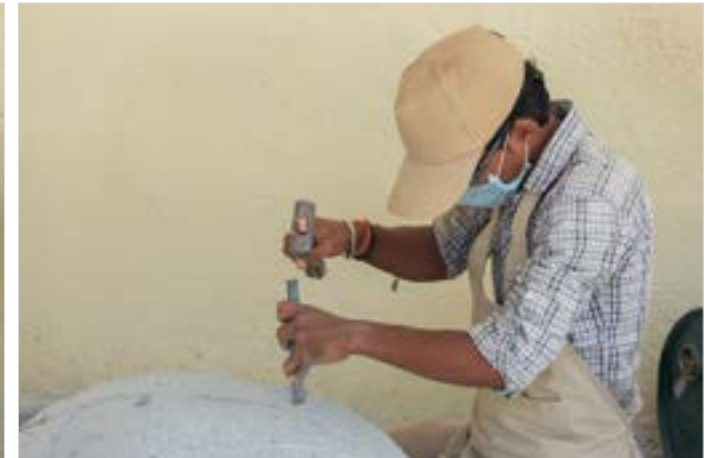
Smoothering the uneven surface using flat chisel.
