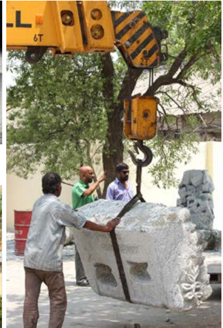
Top and bottom portions are carried individually for the installation.
