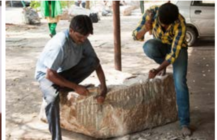
Removing an unwanted stone by striking chisel.
