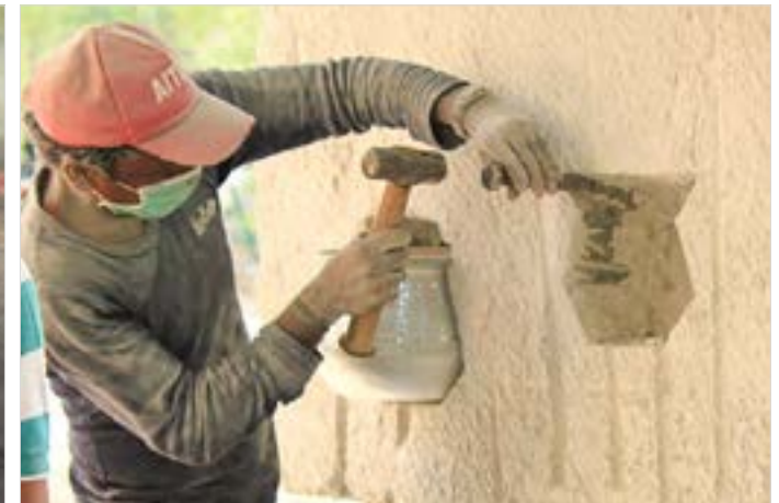
As per the marking the stone is roughly carved.
