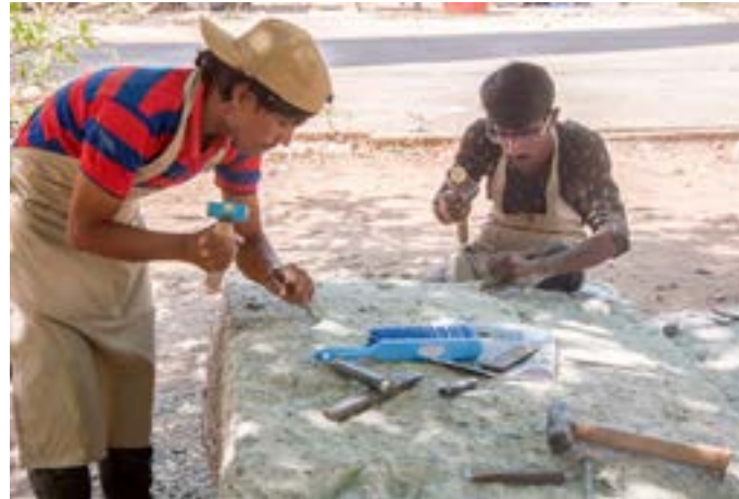
Later the stones are laid horizontally and the work gets begin.
