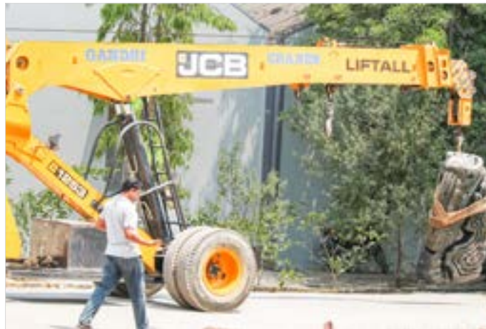
Then the sculpture is carried to the installation place.
