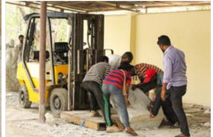
Stone is being carried to the installation site.
