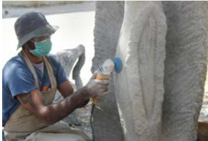
Hand buffing machine is used to smoothen the rough surface.
