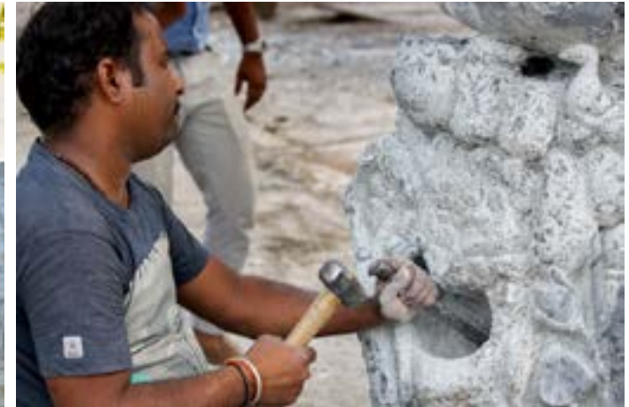
Chiseling out the excess of stone to make it hollow.
