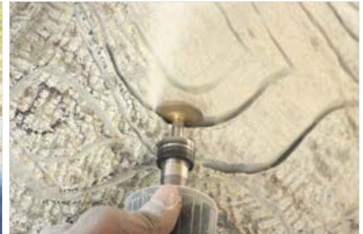
Using die grinder tool, designer cuttings are made.
