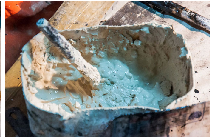
Wood putty is used to fill the cracked surfaces.
