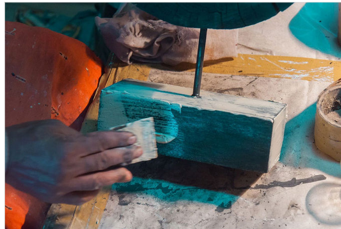
Using a small plywood sheet, putty is applied and smeared to the wood surface.
