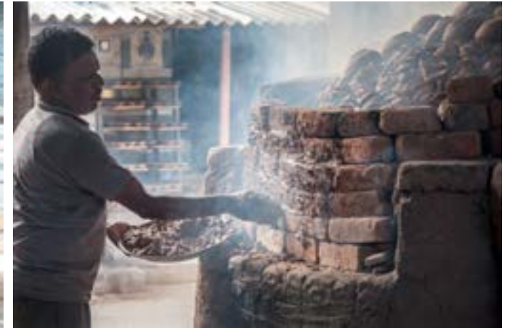
The gap between the bricks are closed with clay.
