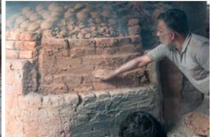
The gap between the bricks are closed with clay to avoid heat dissipation.
