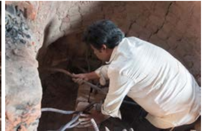
Arranging the iron rod as a base for baking process.
