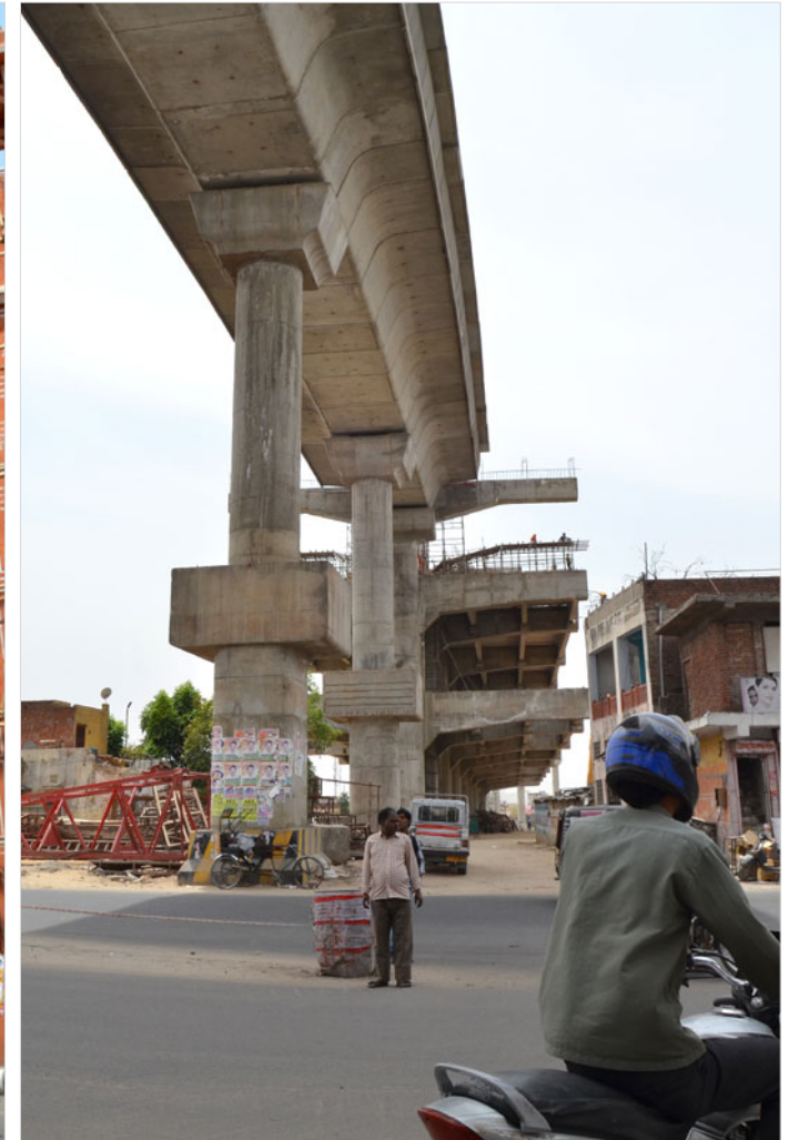
Metro construction in the city.
