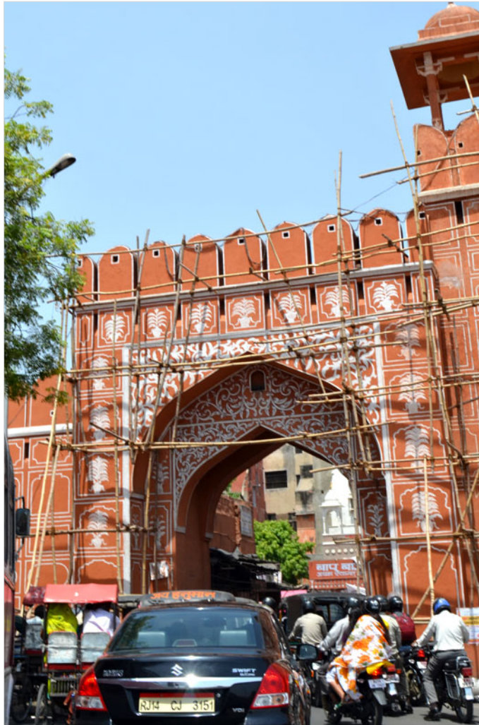
Restoration in progress.
