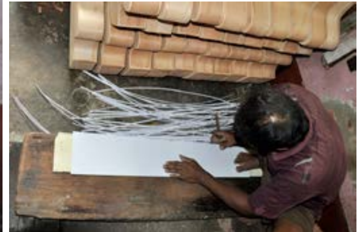
The Decolam sheet is cut into lengthier strips as per requirement.
