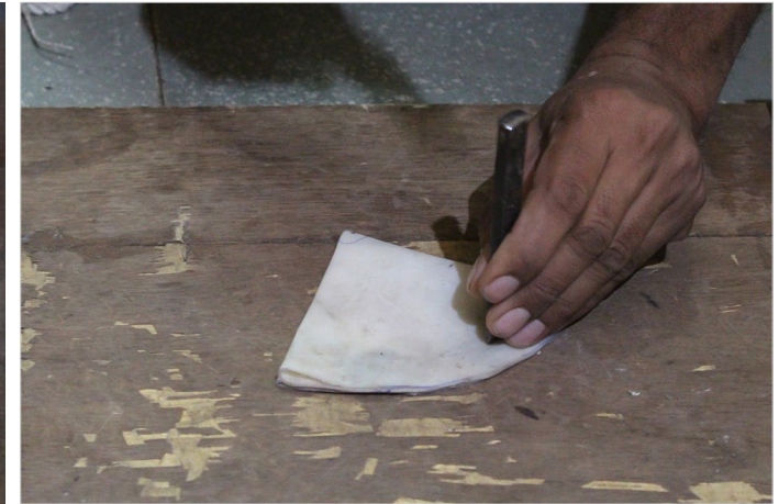
A series of holes being made with a chisel and hammer.
