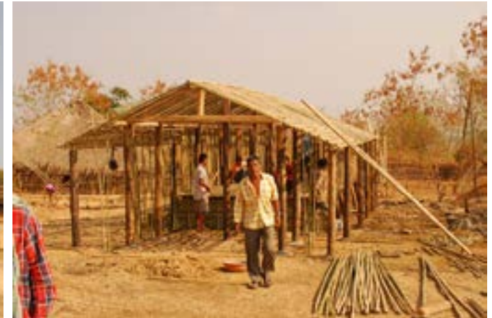
Hut structure from North-East India is been created.
