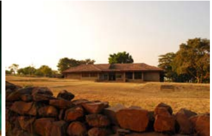
Temporary exhibition hall.
