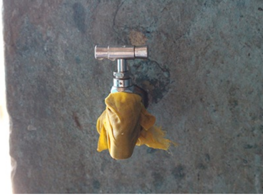
Figure.4 A local household solution to filtering sediment from water is placing a scrap of cloth over the tap.
