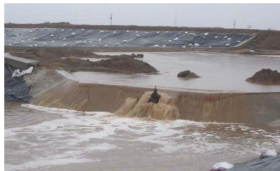
Figure 4: Surface runoff carrying huge silt
