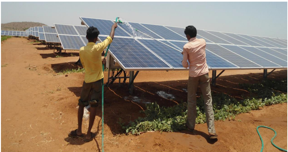
Figure-4: Dual use of water for solar panel wash and irrigation of agriculture produce
