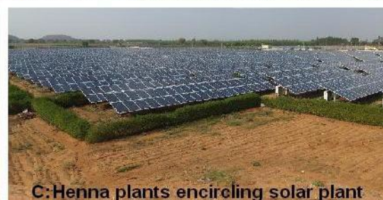
Figure-8: Wind & dust protection of solar panels by creepers and henna plants
