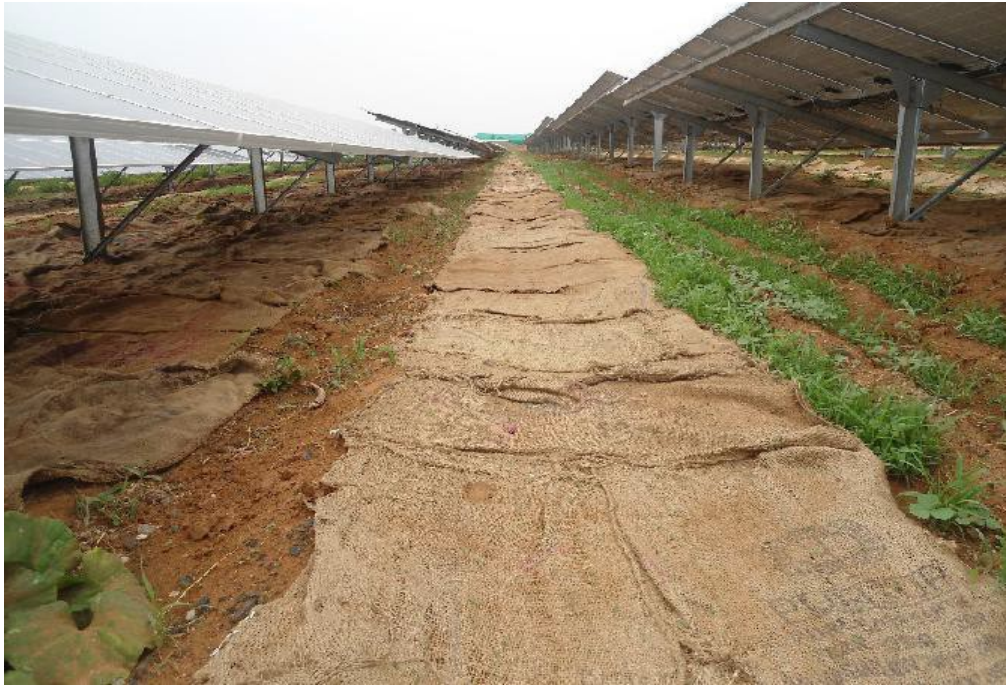
Figure-5: Water retention on land by jute bags.
