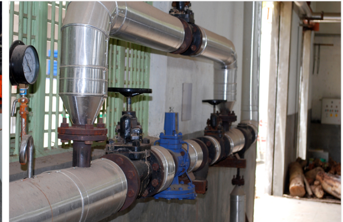
The pipe hose enables the transportation of heat for processing the cocoons.
