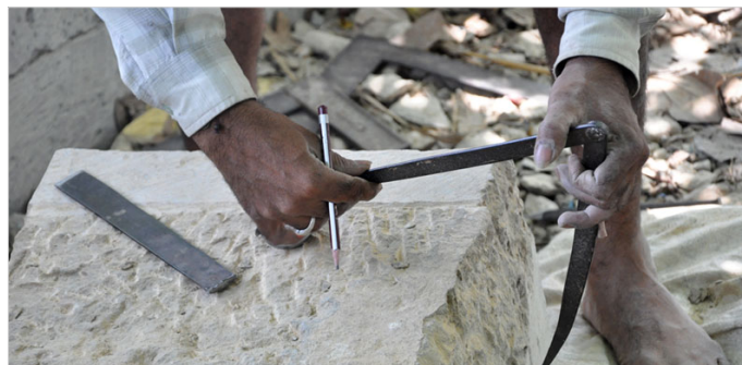
Dimensions are marked with the help of compass.
