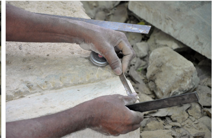
Artisan measuring the length of the stone using tape.
