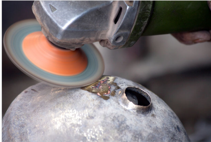
The excess metal is removed after welding.
