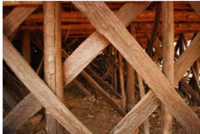
Wooden structure beneath the hut.
