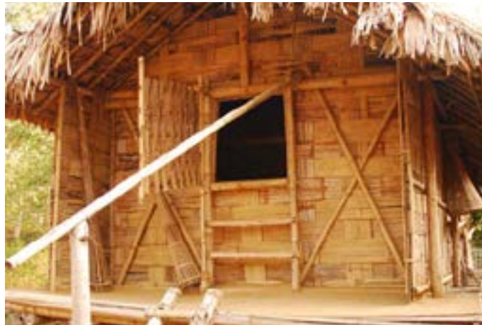
Grain storage room.
